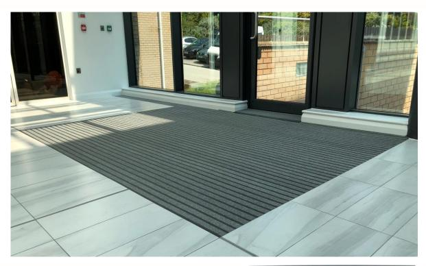
Reference: Access Click Primary Barrier Matting Module: PVC-u base incorporating carpet wipers Construction: Closed Wiper material: Loop pile - 100% Polypropylene Total height (including carpet pile): 12mm PVC-u base height: 10mm PVC-u base colour: Black
